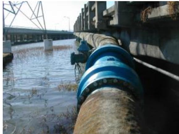
**Steel Pipe with Dielectric Coating, Concrete Armor Shield and Cathodic Protection on Buried Sections. No Sign of Deterioration After 55 Years of Service.**
