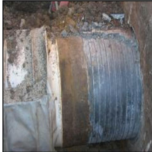
**Detail of Steel Pipe to Concrete Connection
