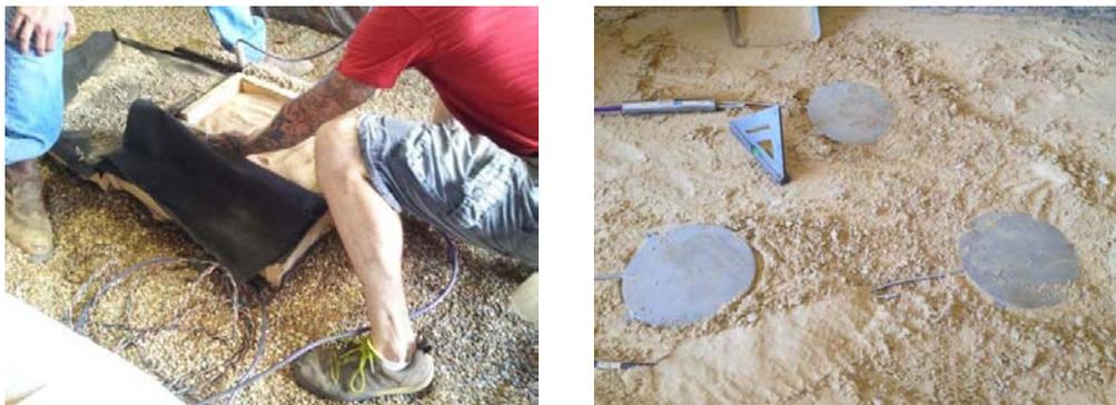
**Figure 5: Placing of the EPCs above the pipe – Pea Gravel (left) and Sand (right)**
