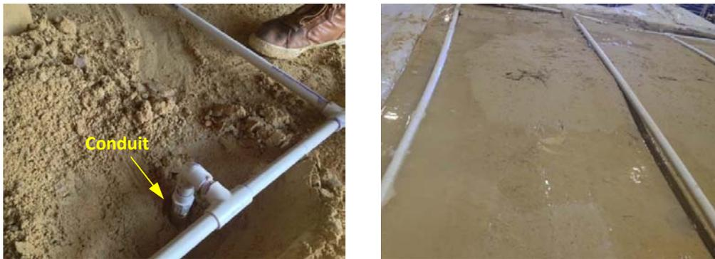
Figure 7: Water Supply Conduit (left) and Perforated Conduits Lying on Top of Soil (right)
