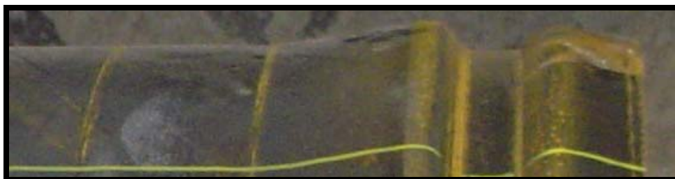
Figure 7 Typical Rolled Groove Shape
