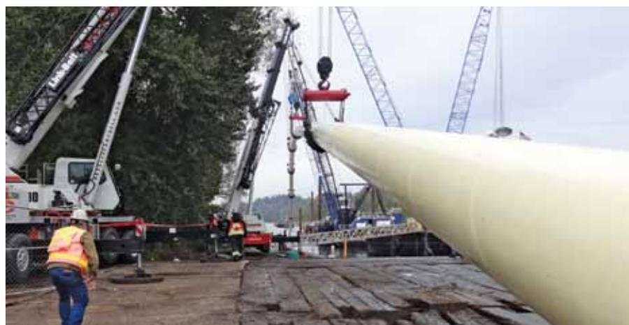
**Pipe is lifted into position for an installation in Lake Oswego, Ore., for the Lake Oswego-Tigard Partnership Project. The project involved a river crossing that was performed via directional drilling for 3,800 ft of 36-in. steel water pipe.**
