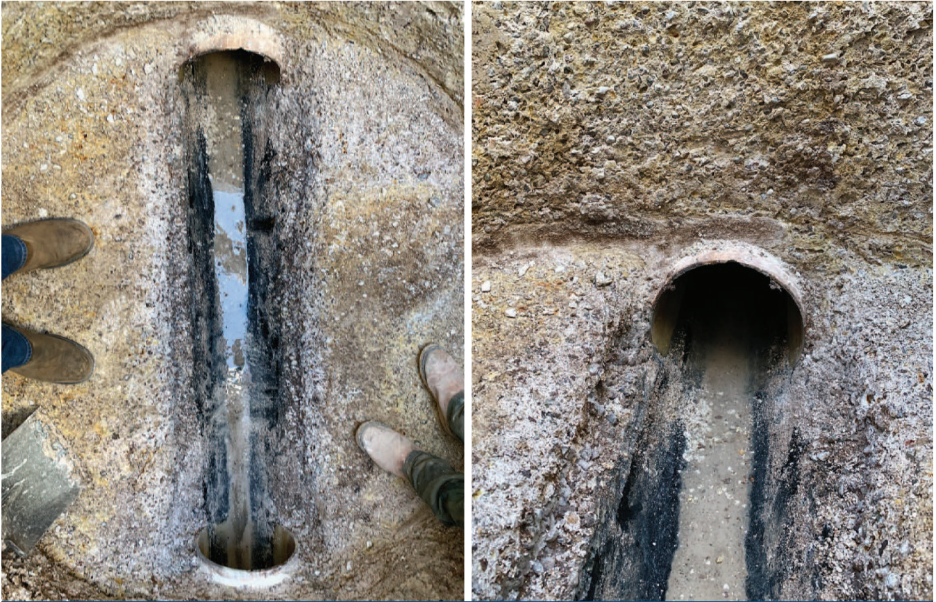
Partially remove bench and channel material (min 2”); clean and remove excess material
