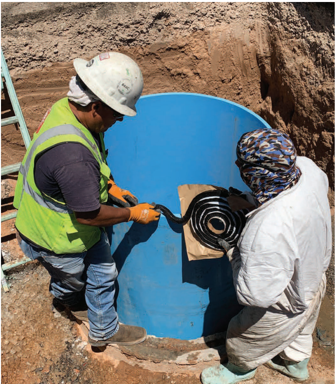
Place butyl rubber sealant on top end of riser
