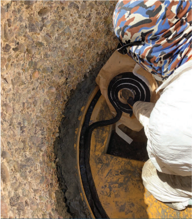
After grout has hardened, place butyl rubber sealant around joint
