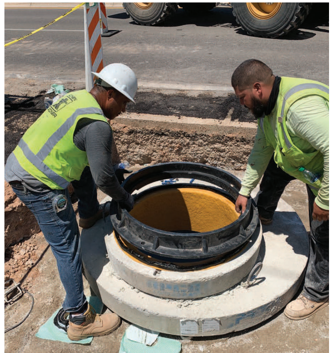
Set manhole cover frame
