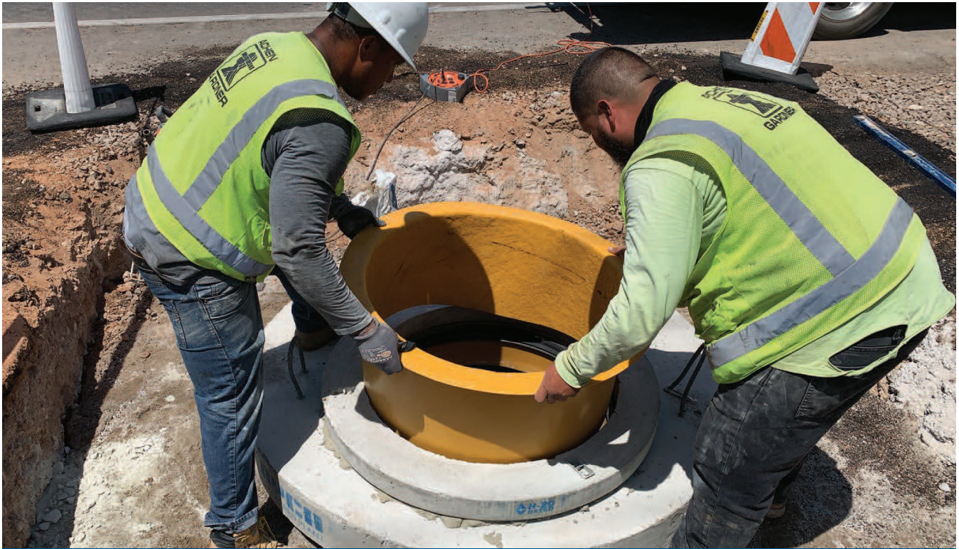
Insert Telescopic Access Collar tube
