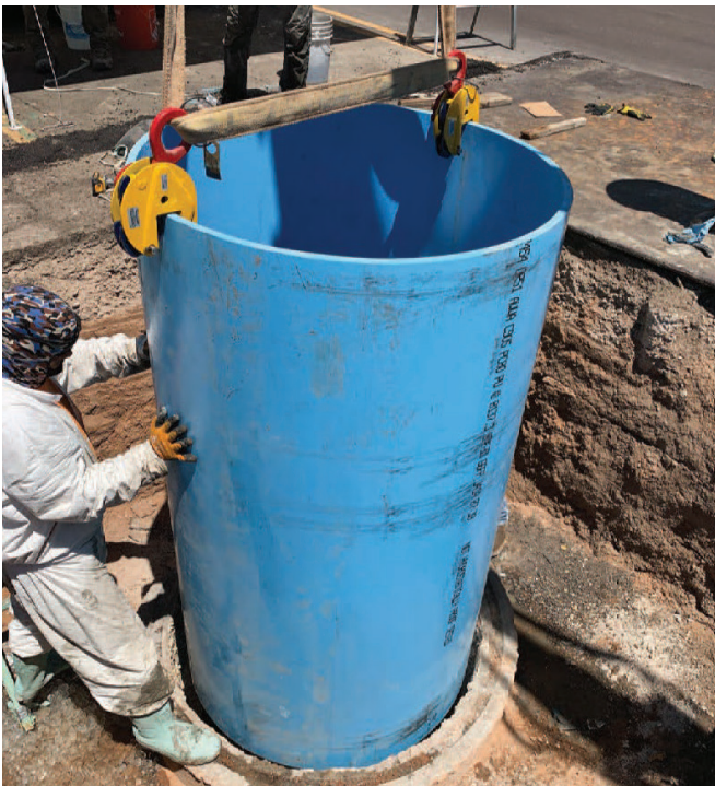
Lower PVC riser into manhole
