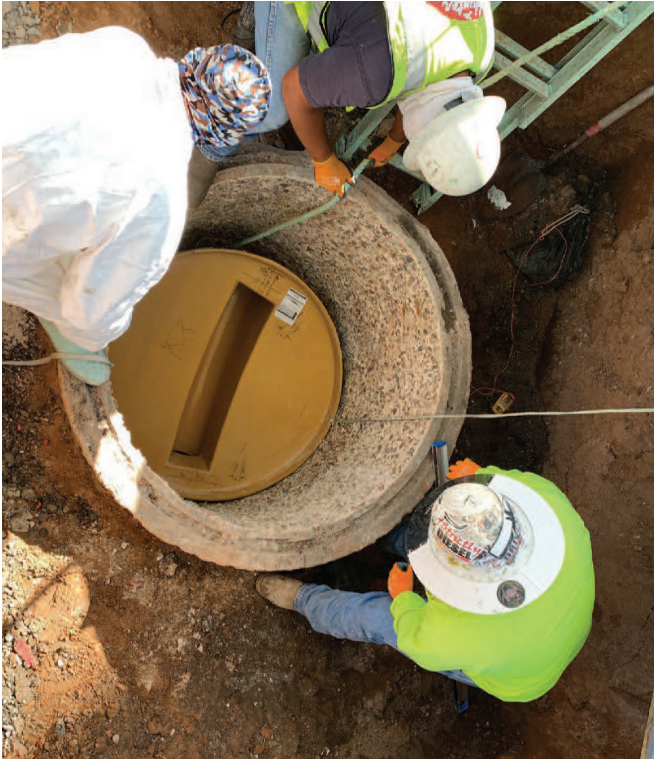
Lower base liner insert into manhole
