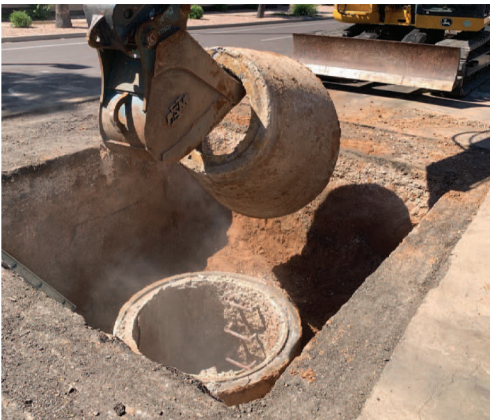
Excavate and remove existing flat top or cone top
