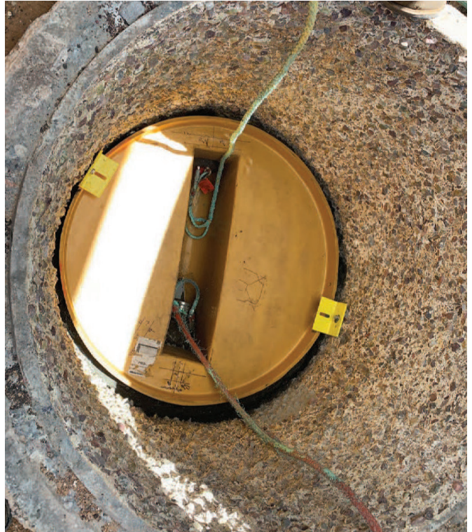
Secure liner in place
