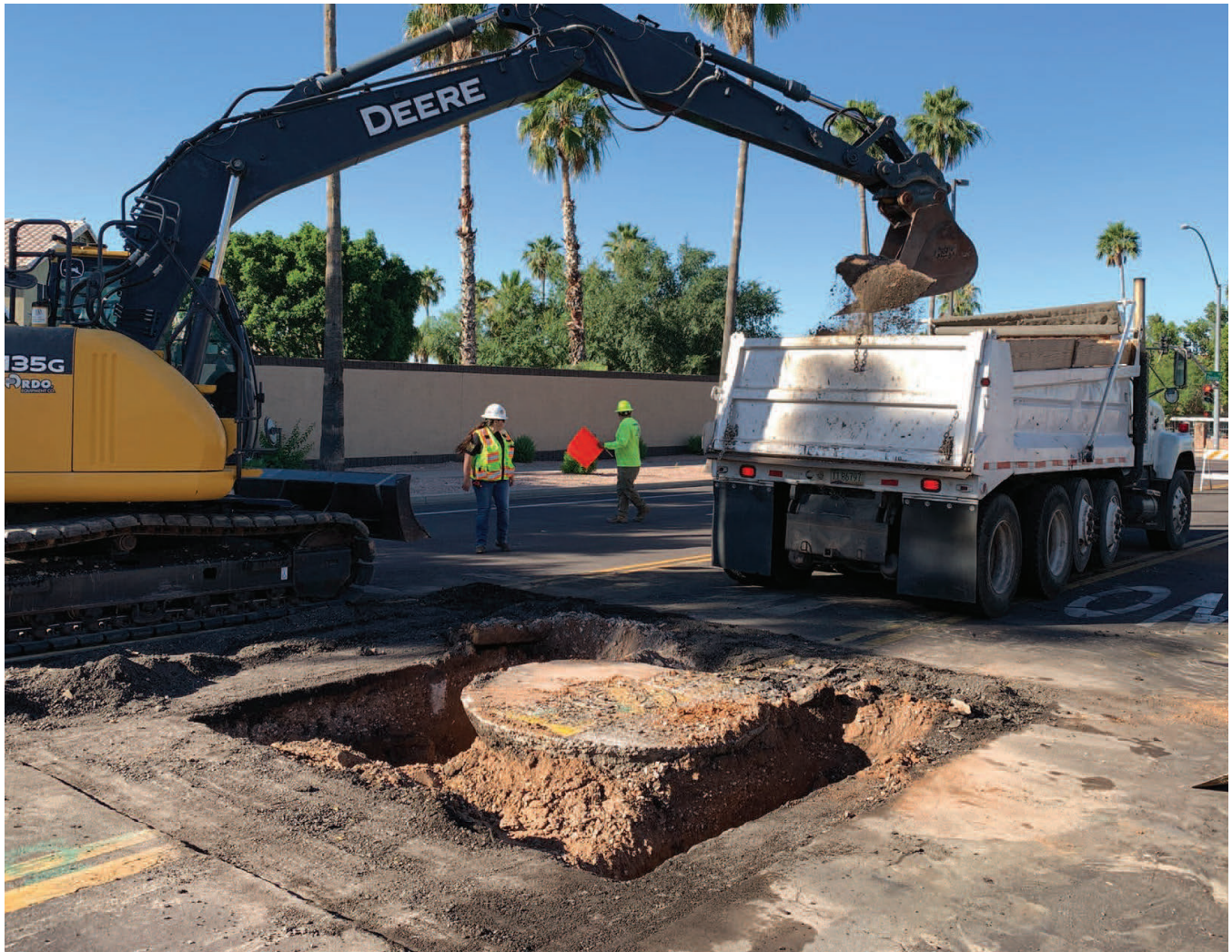
Excavate and remove existing flat top or cone top
