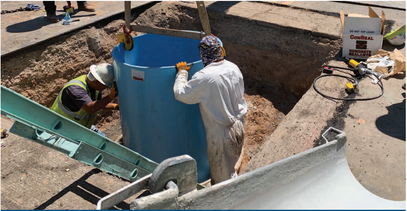
Ensure riser is plumb
