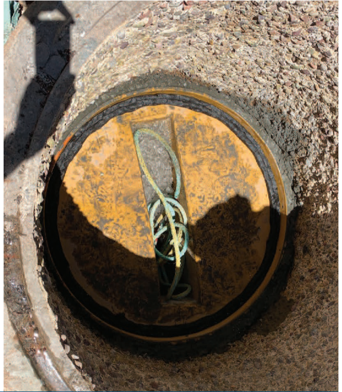
After grout has hardened, place butyl rubber sealant around joint
