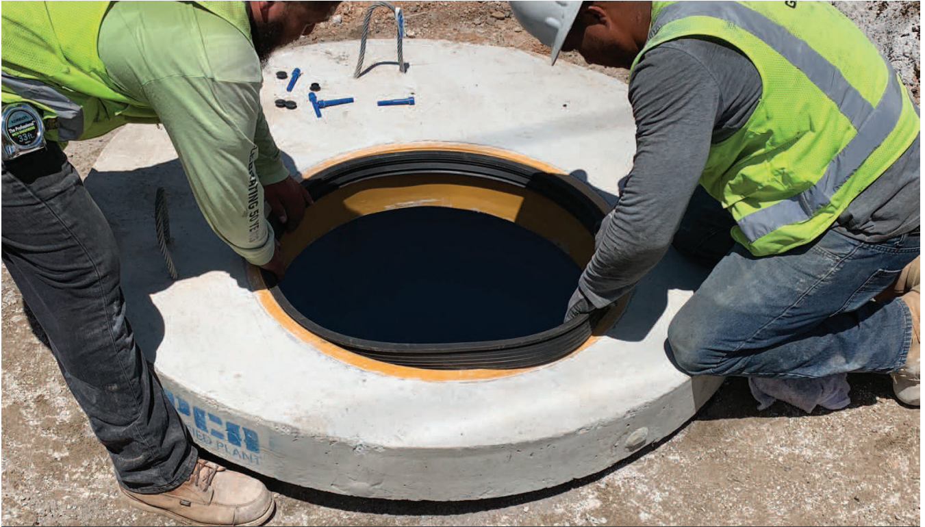
Insert Telescopic Access Collar (TAC) gasket
