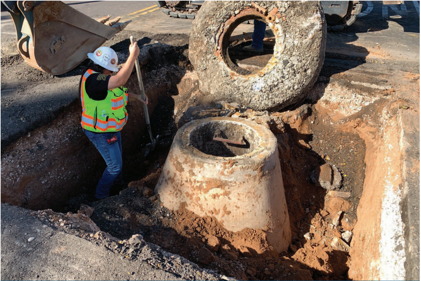
Excavate and remove existing flat top or cone top
