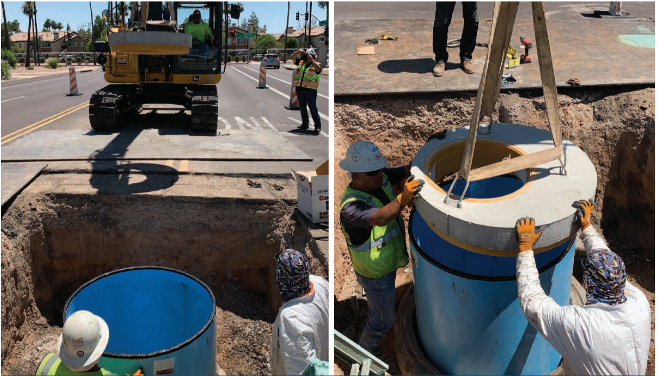
Lower FRP-lined precast lid onto riser
