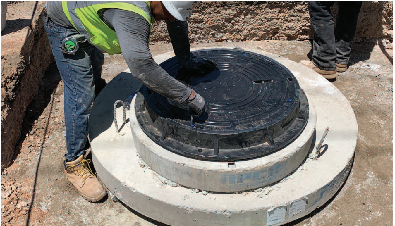
Completed installation (covered)
