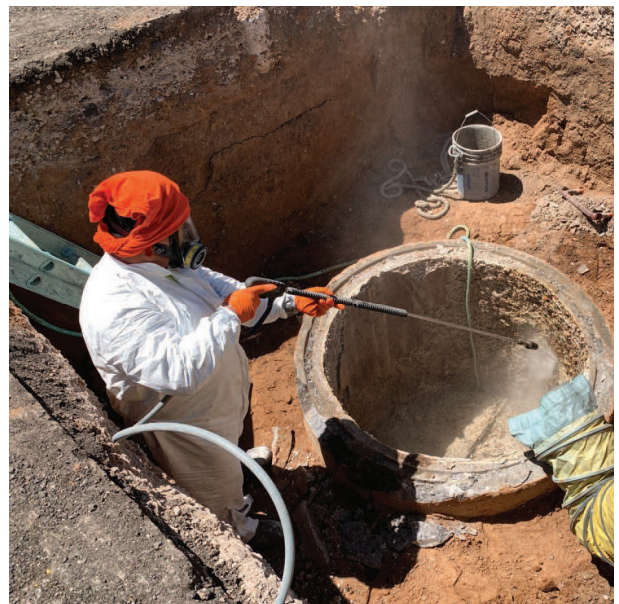
Clean all MH walls. Substantially remove incontinent concrete material
