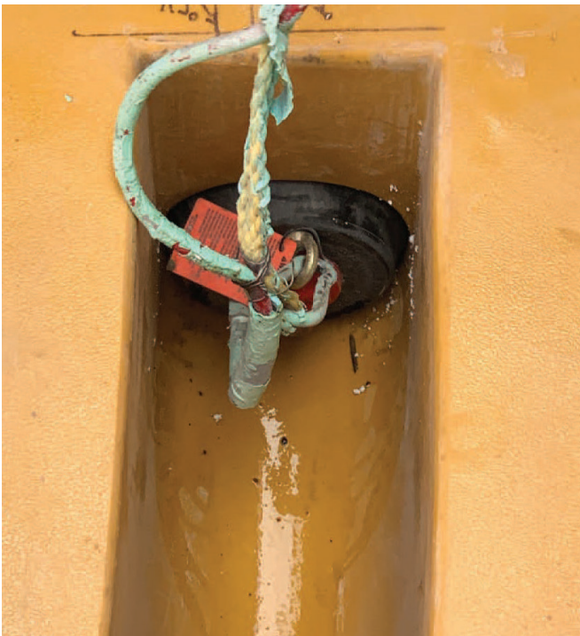
Pipe penetration to be sealed with inflatable plugs
