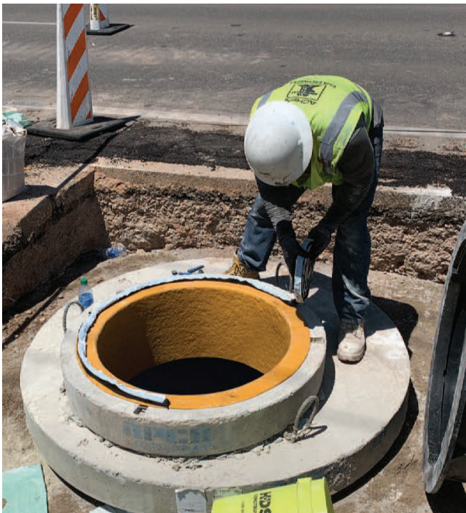
Place butyl rubber sealant on top of flange TAC
