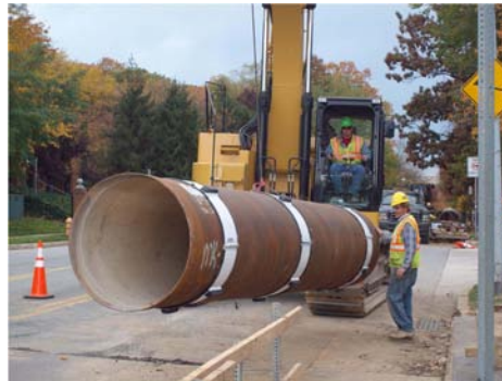
Figures 4a, b: Casing Spacers, 3 Casing Spacers per 20-ft Steel Cylinders
