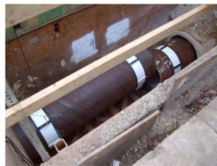
Figures 5a, b: Jacking Machine, Cartridge-Method Insertion
