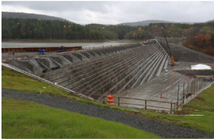
Figure 1. Current Rehabilitated Spillway Control Section at Gilboa Dam
