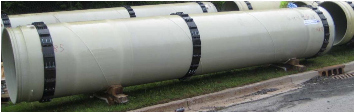
Figure 3: Steel Pipe Liner Sections with Casing Spacers
