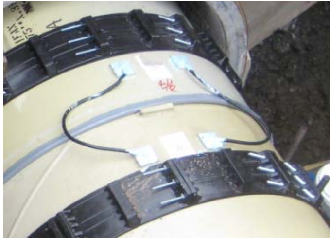
Figure 4: Joint Bonding for Electrical Continuity
