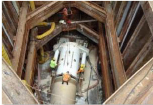
Figure 10. Ala Moana Force Main Project
