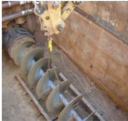
Figure 1. Horizontal Auger Boring
