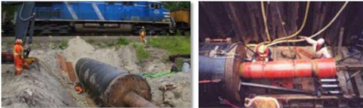
Figure 2. Pipe Ramming
