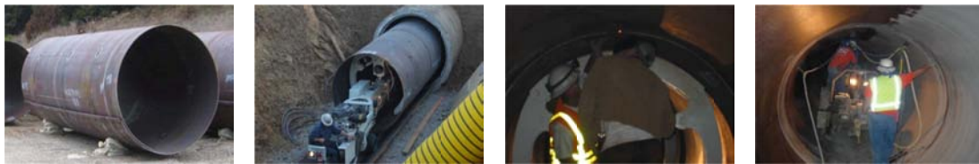
Figure 1a, b, c, d: Collapsed Reliner Cylinder, Insertion of Reliner into Host PCCP, Expansion and Welding of Reliner, In-field Lining Application
