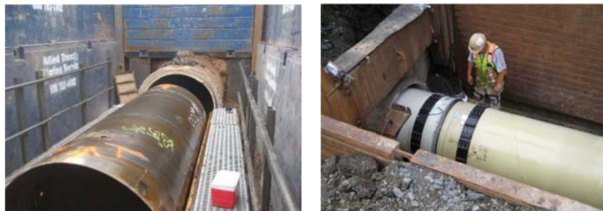
Figure 2a, b: Sliplining 60-inch PCCP in Phoenix, Sliplining 48-inch PCCP in Halifax, Nova Scotia (Bass 2011)
