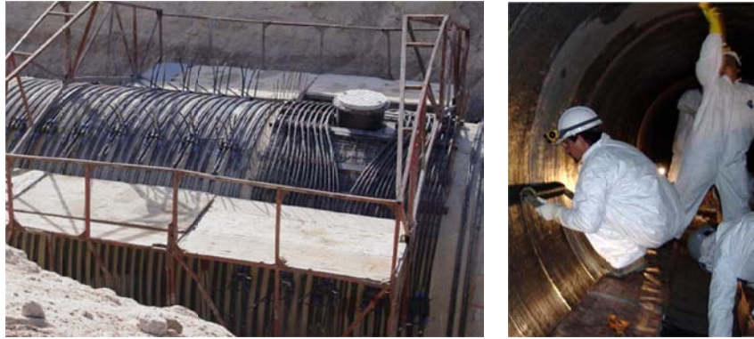
Figure 3a, b: Post-tension Tendon Repair in Libya (Elnakhat 2006), CFRP Application (Rahman 2008)
